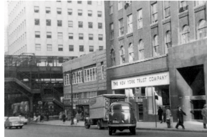
THIRD AVENUE EL DEMOLITION In 1955, the Third Avenue elevated train was removed, opening up opportunities for office development.
