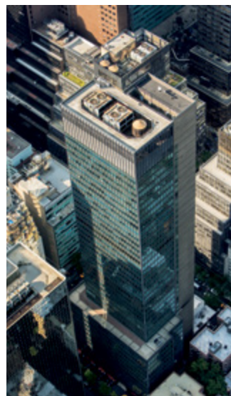
AN AERIAL VIEW Aerial view of 825 Third Avenue outlining the building's proximity to East 50th and 51st Streets. Skypan
